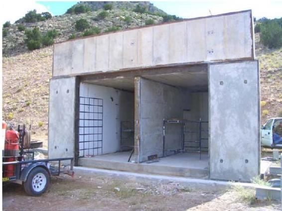
Figure 1. Containment Structure before installation of CMU walls
